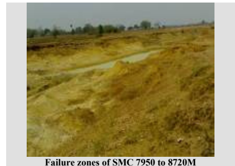
Failure zones of SMC 7950 to 8720M
