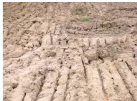
Digging marks of excavator in Bodhi tank at Latar of Ranapur block
