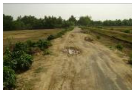
1C1 canal embankment road from Dhoda to Nandipur not providing all weather access after spending Rs 7.26 lakh by Dasarathpur block and overlapping execution by Irrigation Department
