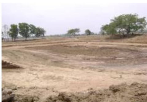
Bodhi tank at Latar of Ranapur block excavated using excavator and tractors
