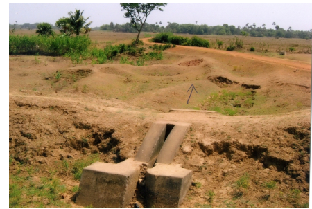
Damaged Manaour minor of Paika Rt distributary
